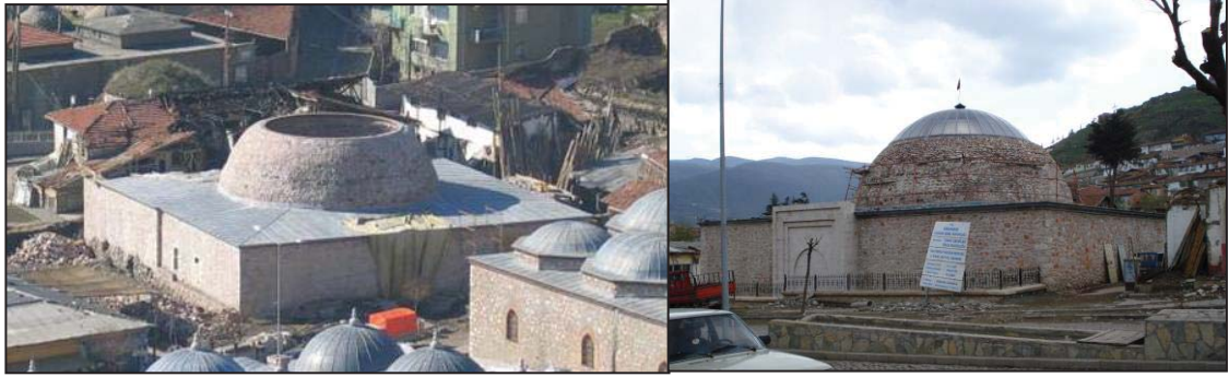
Figure 14 (a, b). View from renovated Çukur Madrasa
