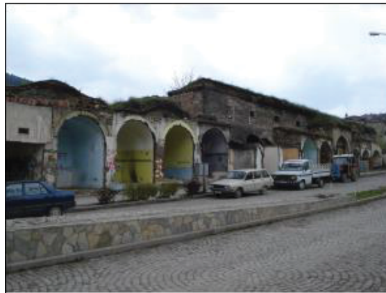
Figure 8. A view from Deveci Inn
