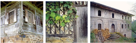
Fig. 14. Outer walls in the vernacular houses (Batur,2005)
