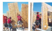
Fig. 11. The installation of SIPs (Morley,2000).
