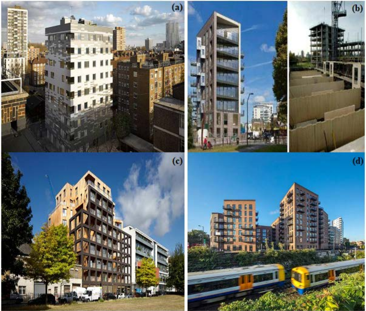
Şekil 25. Murray Grove (a), Bridport House (b), Wenlock Cross (c), Dalston Works (d)
