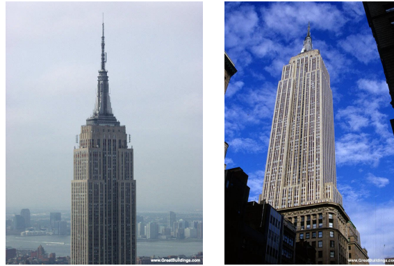
Şekil 133. Empire State Building, Shreve-Lamb-Harmon, New York, 1931
