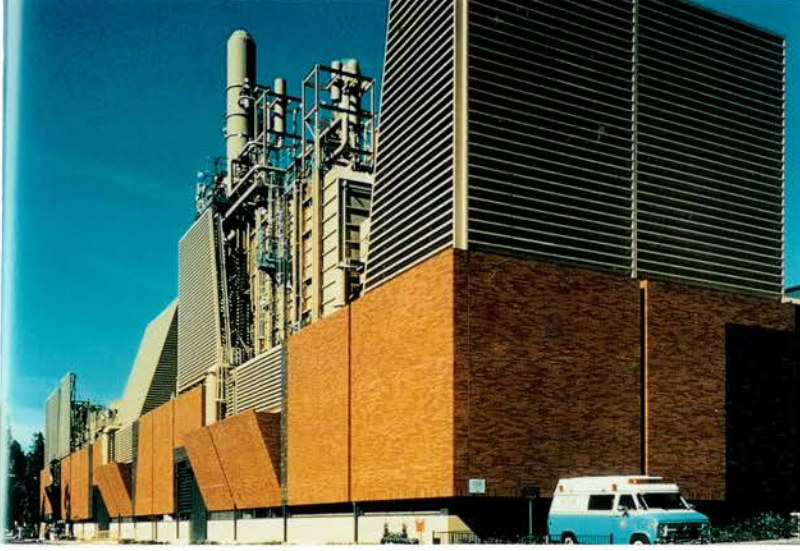
Şekil 18. Ucla Chiller Plant/Facilities Complex
