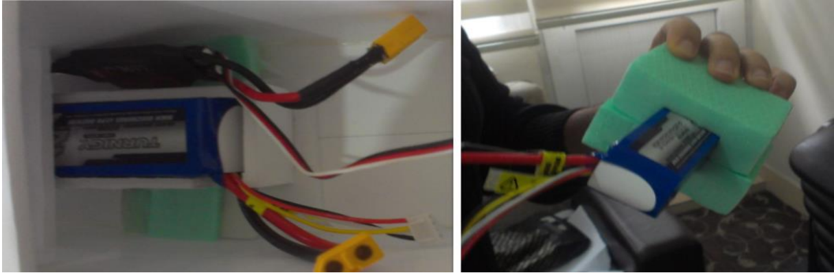
Fig. 6.8 Installation of power system
