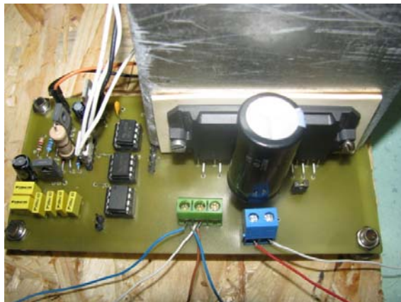
Figure A.6.2. The general view of inverter system
