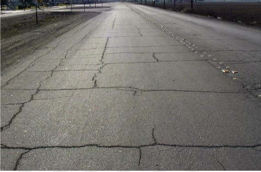
Şekil 8. Termal çatlaklar (California Department of Transportation, 2001).
