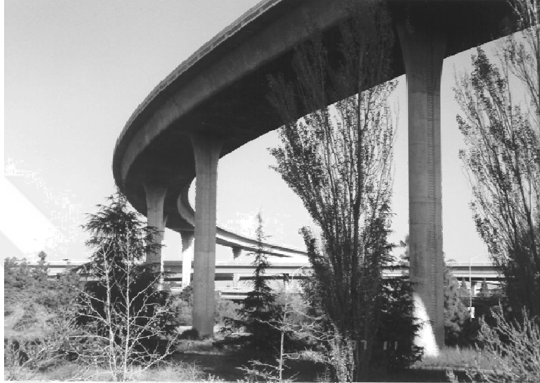
Figure 2.4. Prestressed box-girder bridge (I-280/110 Interchange, CA)
