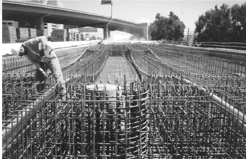
Figure 2.2. A post-tensioned box-girder bridge under construction
